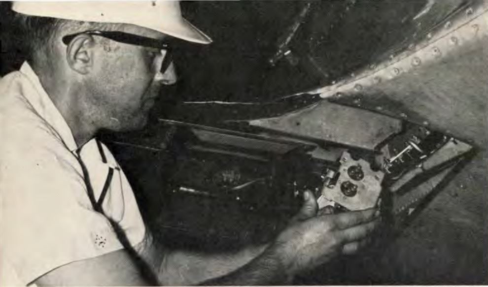
Culprit! Voltage regulators were involved in 12,600 malfunctions and nearly 500 aborts during a six-month period last year.
